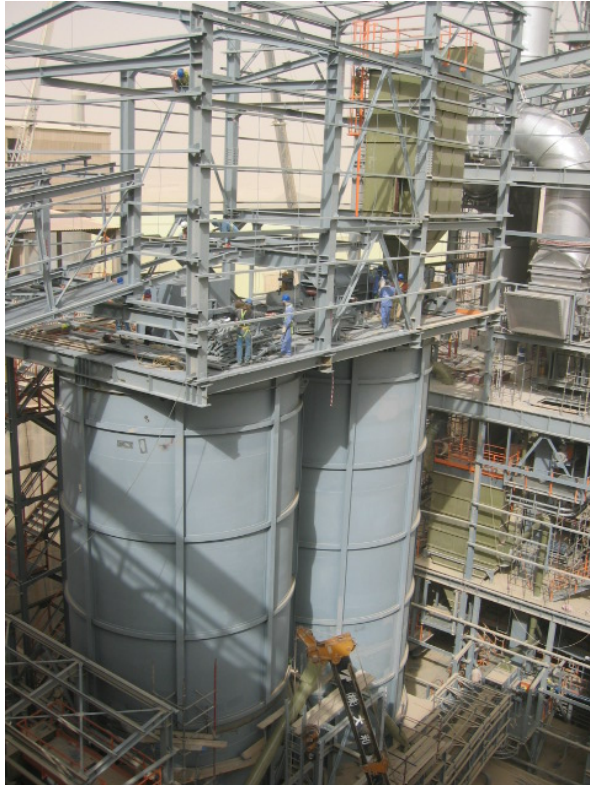
a. During Erection Stage
